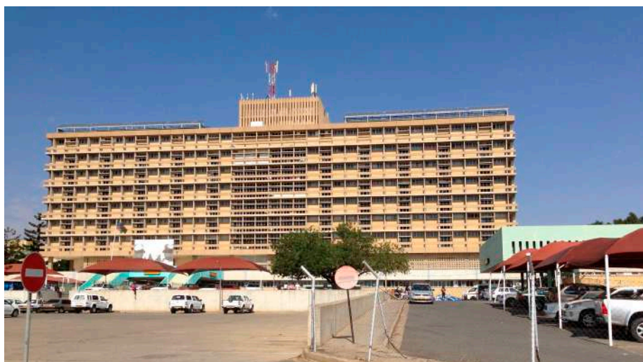
Figure 1. The Windhoek Central Hospital.
